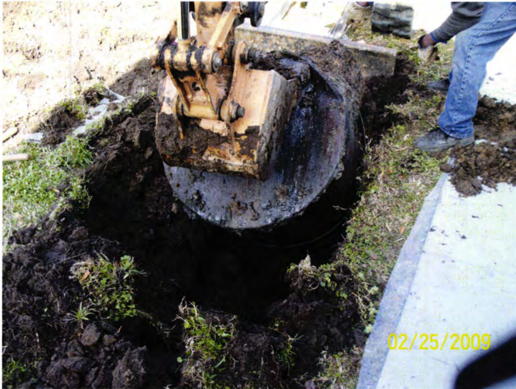
Picture 3: UST 128Banyan-2 being removed from the excavation.
